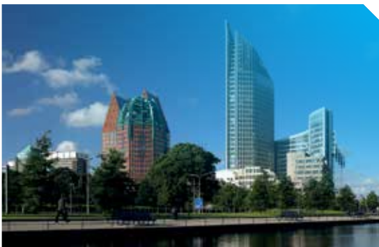
Ampetronic low-spill loops used on twenty nine floors of The Hoftoren, The Hague, The Netherlands
