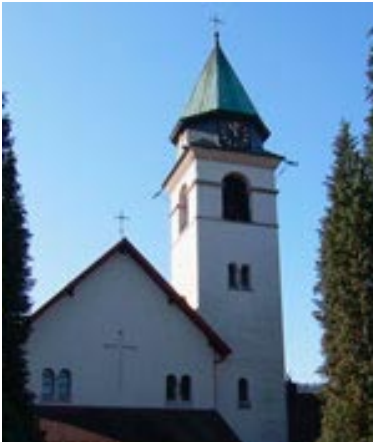
Church with AFILS system installed
